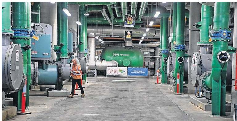
These pipes channel cold water from the harbour through the buildings to keep them cool as an alternative to standard air-conditioning. PHOTO: NICK MOIR
